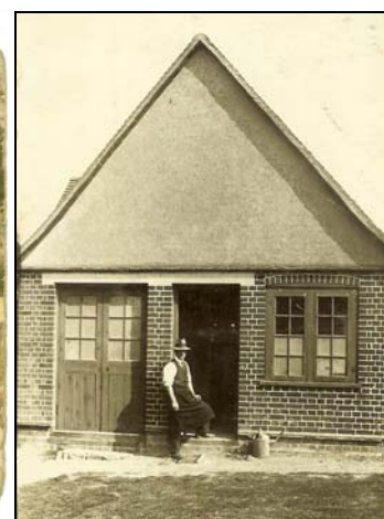
Mrs Doreen Warren's grandfather, Mr Ernest Beaney, working as Head Gardener at Shottendane circa 1920. This boiler-house still stands but the doorway on the right and the window are now sealed up
