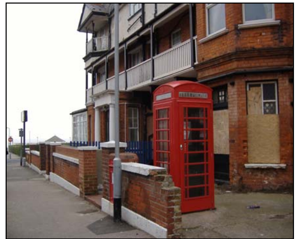
The K6 kiosk in Norfolk Road (2006) before the demolition of the Norfolk Hotel seen behind the kiosk (note that the kiosk is within the curtilage of the hotel site)
