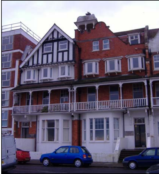
Nos 11 Lewis Crescent (on the right) and No. 12 Lewis Crescent – the two properties formed the Hotel Majestic and are now Majestic Court
