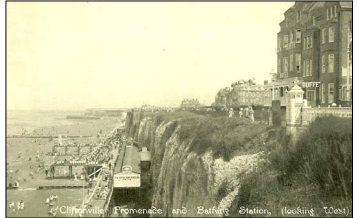
Pettman's Bathing Station below the Queen's Highcliffe Hotel. Newgate Gap Bridge can be seen on the right
